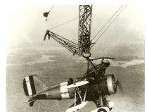
aircraft's hangar deck. The airplanes were released via a trapeze and a harness which lowered the planes through a
