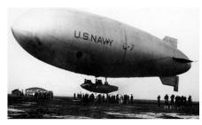
The **C-class blimp** was a patrol airship developed by the US Navy shortly after World War I, a systematic improvement upon the B-type which was very suitable for training, but of limited value for patrol work. Larger than the **B-class**, these blimps had two motors and a longer endurance. In 1921, the **C-7** was the first airship ever to be inflated with helium. First flight 30 September 1918, at Wingfoot Lake; retired 14 Aug 1920, 20 built.
