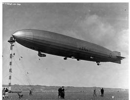
USS Shenandoah was the first of four United States Navy rigid airships. It was constructed during 1922–1923 at Lakehurst Naval Air Station, and first flew in September 1923. Shenandoah was originally designated FA-1, for "Fleet Airship Number One" but this was changed to ZR-1. The airship was 680 ft (207.26 m) long and weighed 36 tons (32,658 kg). It had a range of 5,000 mi (4,300 nmi; 8,000 km), and could reach speeds of 70 mph (61 kn; 110 km/h). Shenandoah first flew on 4 September 1923.
